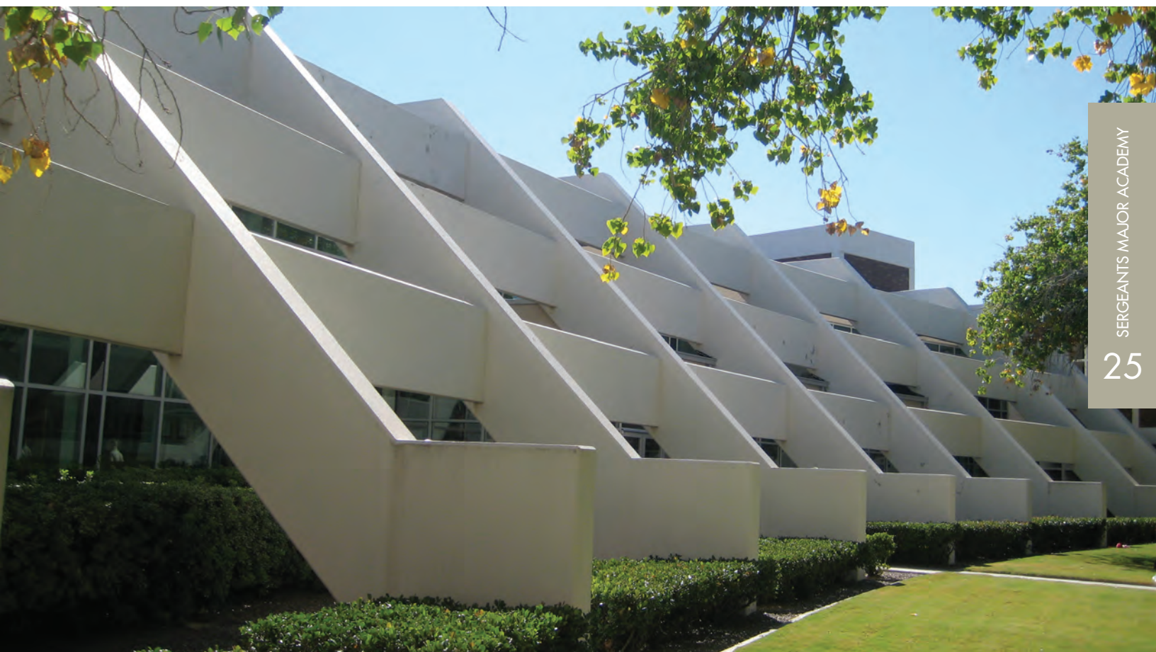
Buttresses on the west elevation of the 1997 East Classroom wing.
