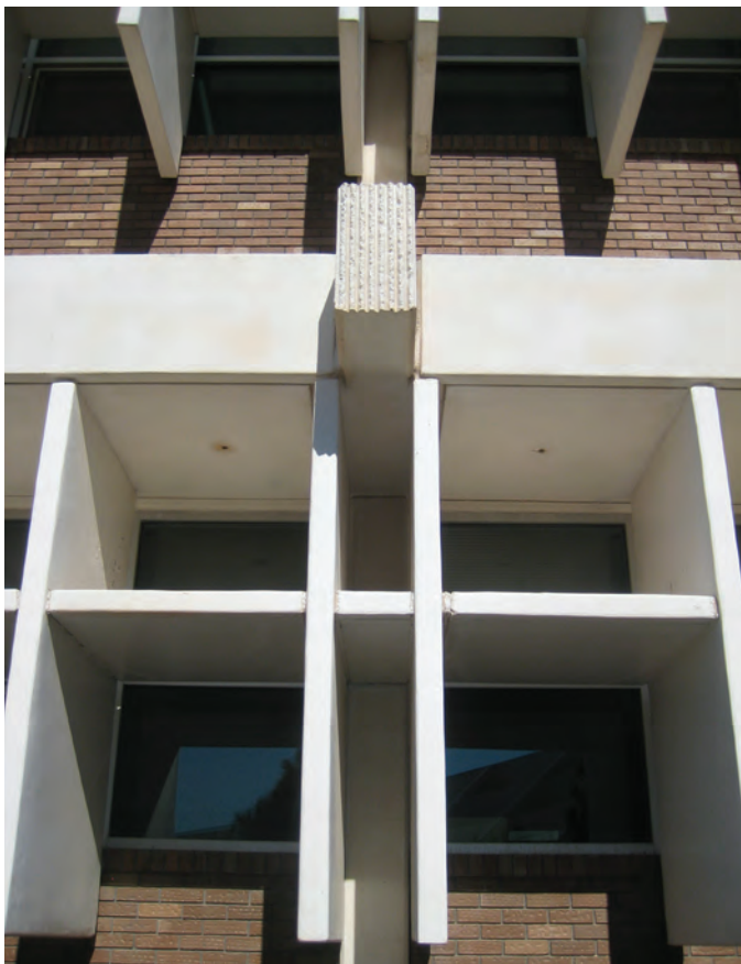
(Above) South elevation, North Classroom Wing. Shelves (horizontal elements) and baffles (vertical elements) form the daylighting system around many of the windows at the Sergeants Major Academy. (Below) Shelf and Baffle Detail, south elevation, North Classroom Wing.
