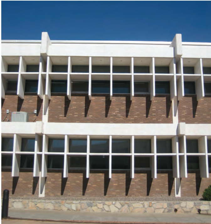
(Above) South elevation, North Classroom Wing. Shelves (horizontal elements) and baffles (vertical elements) form the daylighting system around many of the windows at the Sergeants Major Academy. (Below) Shelf and Baffle Detail, south elevation, North Classroom Wing.
